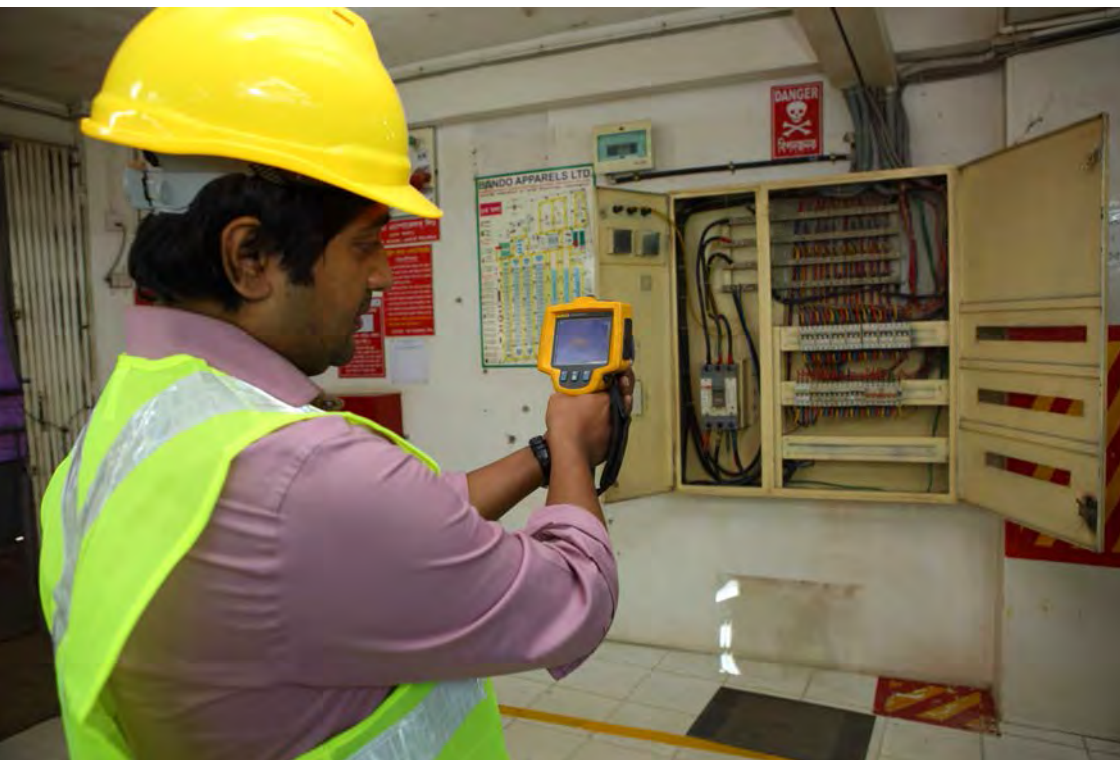
An engineer checks electrical safety in a ready-made garment factory.
